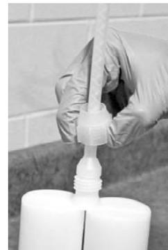
2. Place the Injection Resin dual cartridge in to the manual dispensing tool. Remove the plastic cap and then twist and pull to remove the plastic seal. Replace seal with restrictor, place the 1/4 X 24 mixing nozzle on top of restrictor over the end of the cartridge attaching with the plastic nut.
