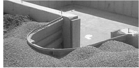
Installed Modular Well
