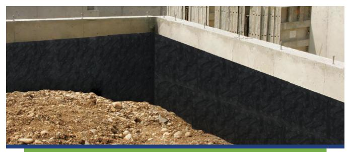
GeoMat "C" Drain 110 and "C" Drain 150 Drainage Boards provide commercial buildings with high-flow drainage protection and a high compression rate.
